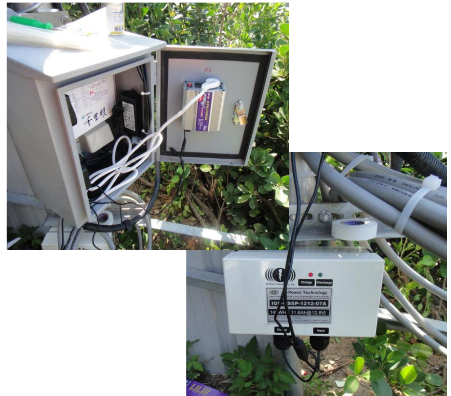
4. Street lamps DC UPS power system and 12VDC to 110VAC converter & optical transponder install images, total install 14 Unit Street lamps DC UPS for Point 1 ~ Point 16
